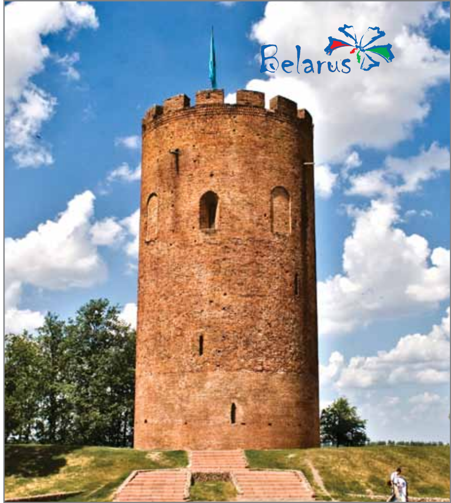
▲ Kamenets tower is one of the best-preserved defensive towers on the territory of the Eastern Europe and the highest one (about 31 m).
